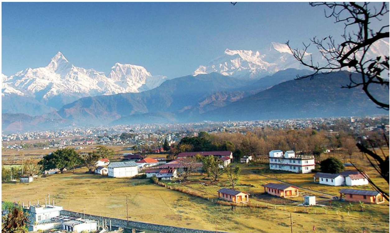
The Green Pastures Hospital and Rehabilitation Centre complex where PSC is located
